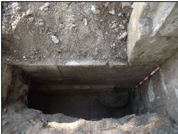
FOTO 3. Contrafort 1. Vessant oest.
